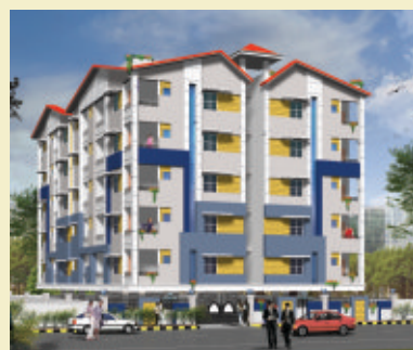
Siri Residency at Hi-Tech City
